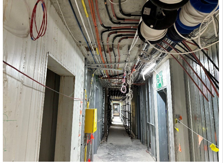
Photo 8: Internal services fitout
