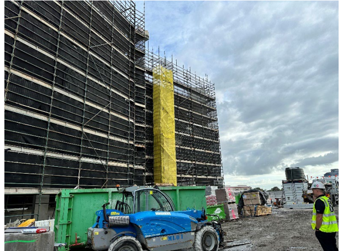
Photo 2: General Construction and dust Shade cloth
